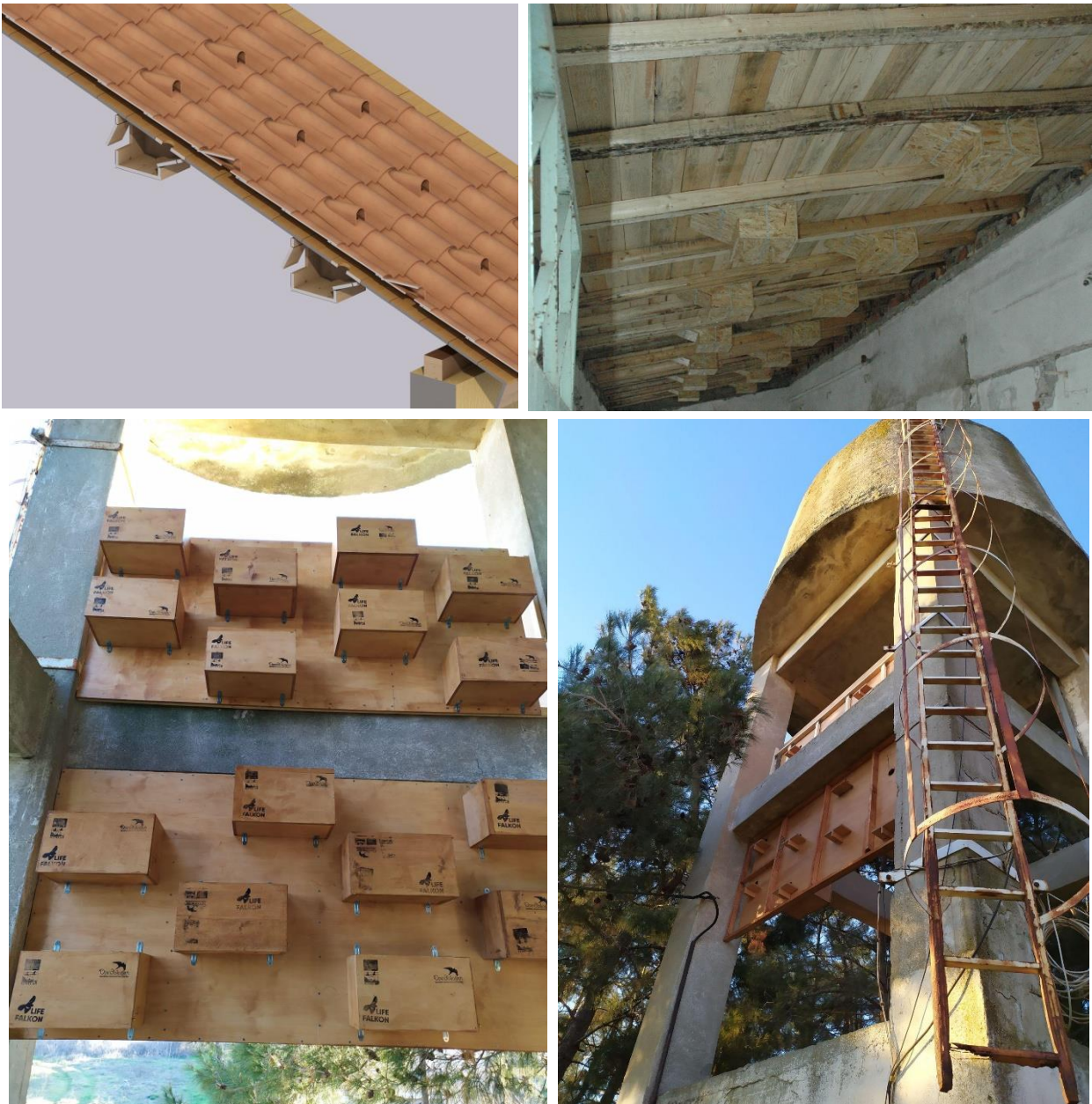
Figure 9. Above: architectural cross-section and photo of wooden nestboxes installed under roof - inside a building. Below: Wooden nest complex (wall type) constructed in the PA of Komotini, Greece (inner and outer views).
